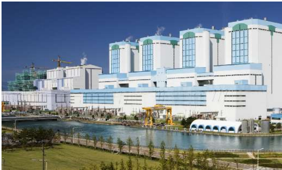
Power Plant : CWP, COP, BFP, GSP, Sump
