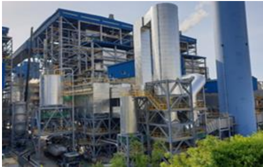
Hyundai Oilbank #3,9,10 Desulfurization Facilities
