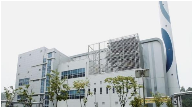
Municipal Waste Incinerator Facility
