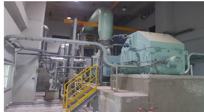
Turbine Installation Construction
